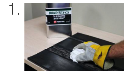
1. Thoroughly clean the working surface
