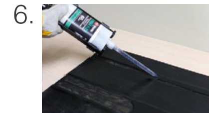
6. Apply Permaflex repair material
